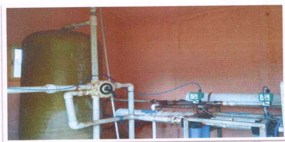
RO Water Unit Inside the campus
